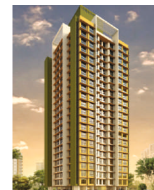
ADITYARAJ AVENUE VIKHROLI
