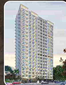
PRAGATI REVANTA BLDG. 48 GHATKOPAR (E), MUMBAI
